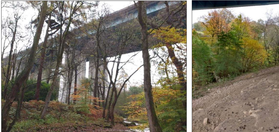
Figures 8.5 and 8.6: Sparse tree growth and poor ground cover around and under the viaducts at Stanworth Valley woodlands
