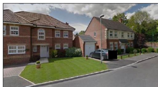
Figure 7.9 New housing off Deadmans Lane
