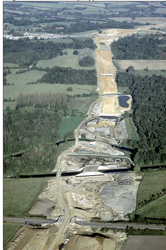
Figure 1.2: Newbury Bypass construction
