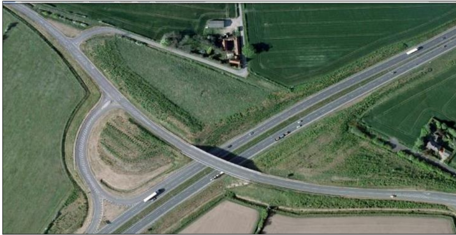
Figure 9.7: Aerial view of Colton’s Farmhouse (top centre of picture) showing proximity of overbridge and embankment
